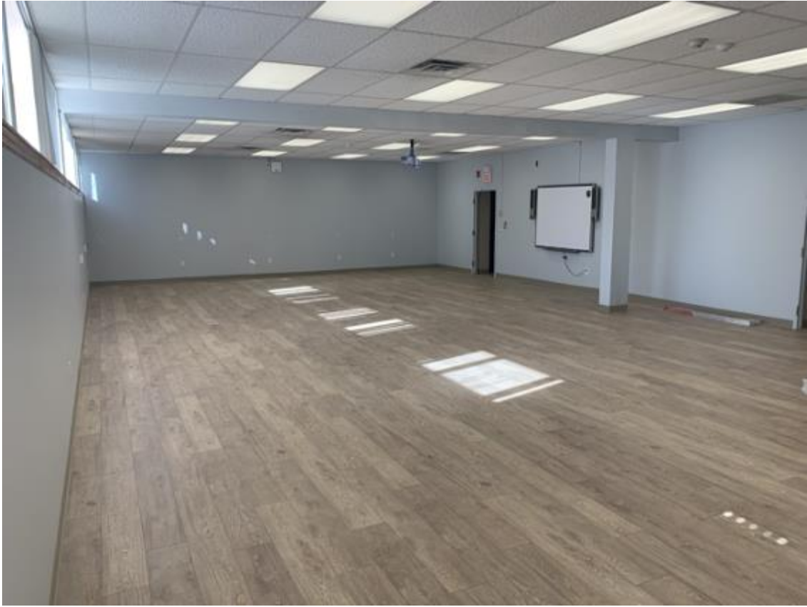
EH K of C Lounge - Completed Beautiful Laminate Flooring
