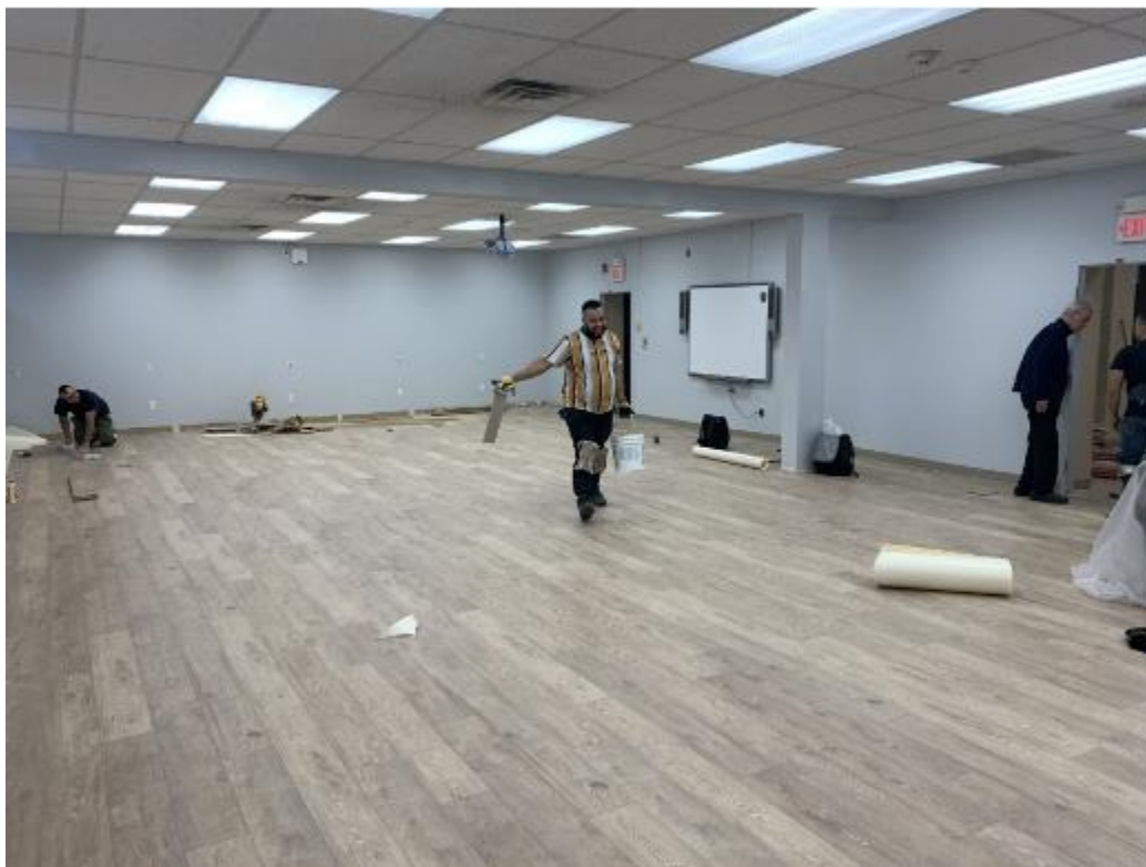
Luxury Floors Installer Working Hard
